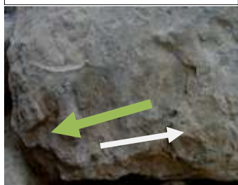
Fig. (8) Exfoliation of the engraving limestone in Abu Musa Excavation.
