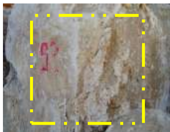
Fig. (5) Crystals of soluble salts pushing off a surface layer of stone.
