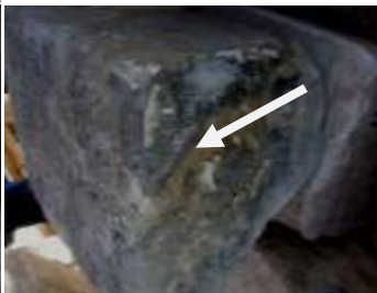
Fig. (12) Black rust found in the surface of some limestone blocks.
